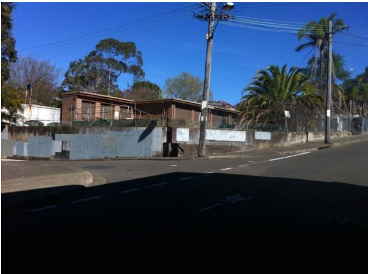
Photograph 2: 35 Edna Street, Lilyfield as viewed from Piper Street and White Street looking south west.
