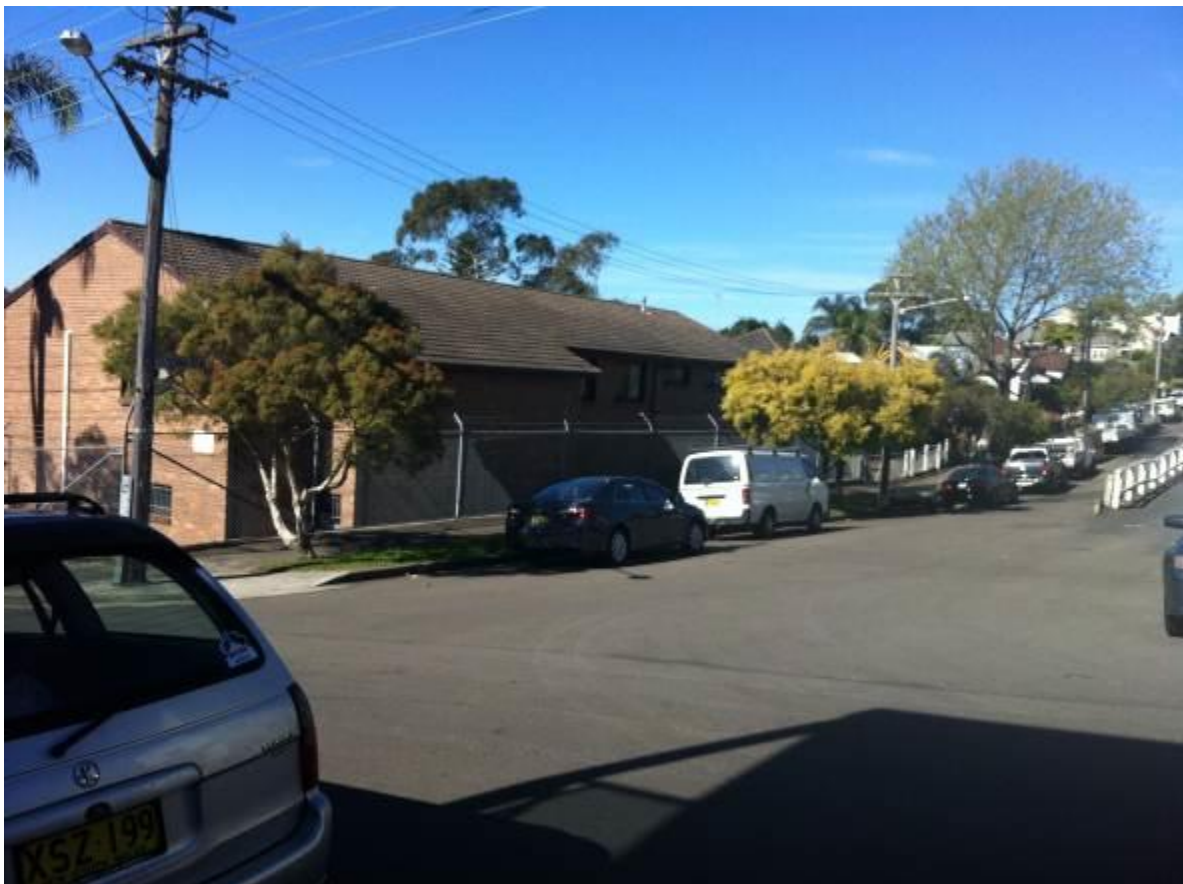
Photograph 4: 35 Edna Street, Lilyfield from corner of Edna Street and Piper Street looking south east.
